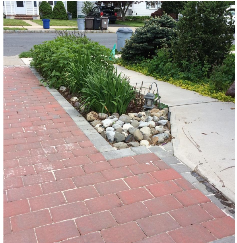
Installed Rain Garden
