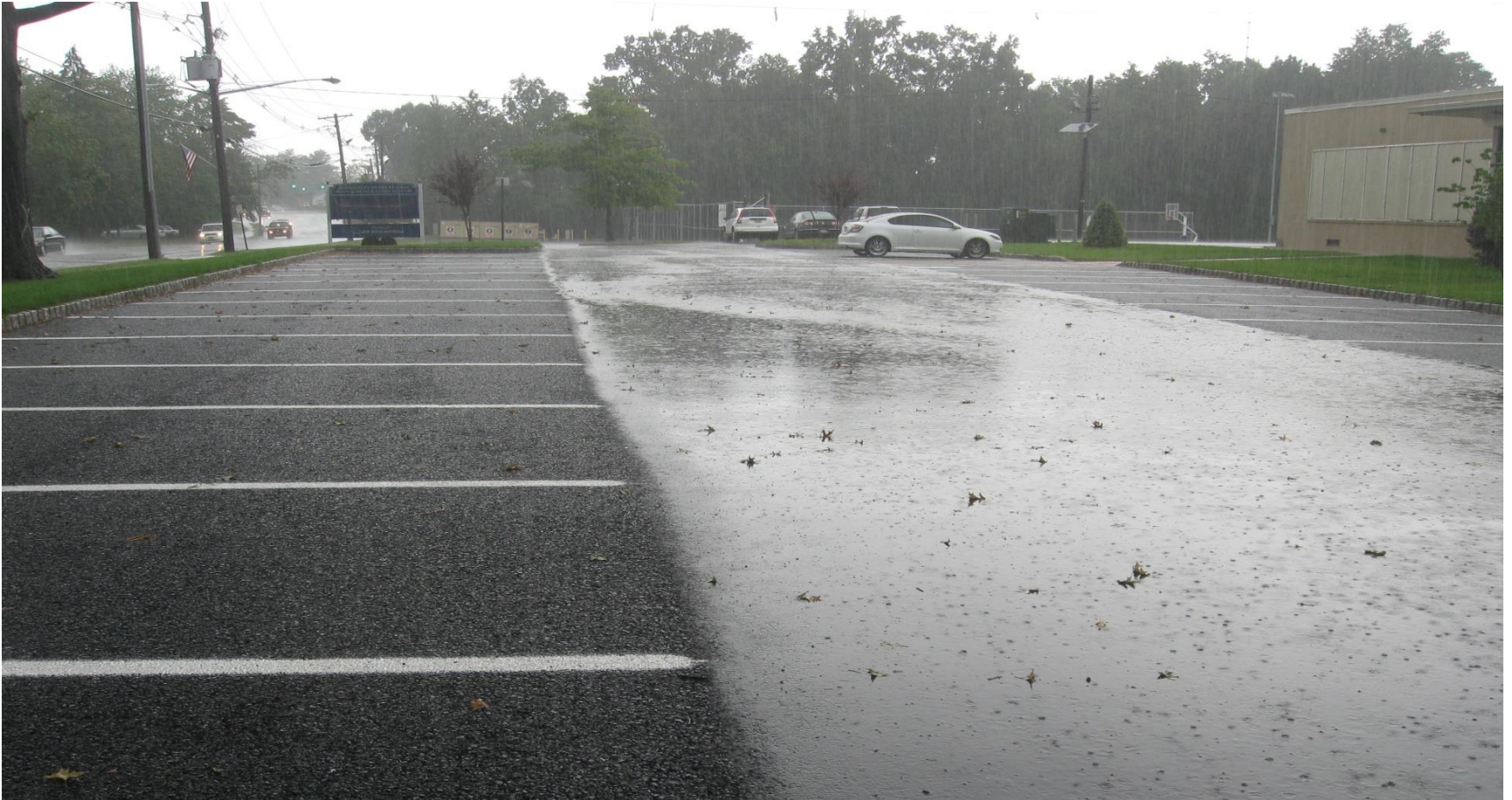
Porous Asphalt Parking Lot
