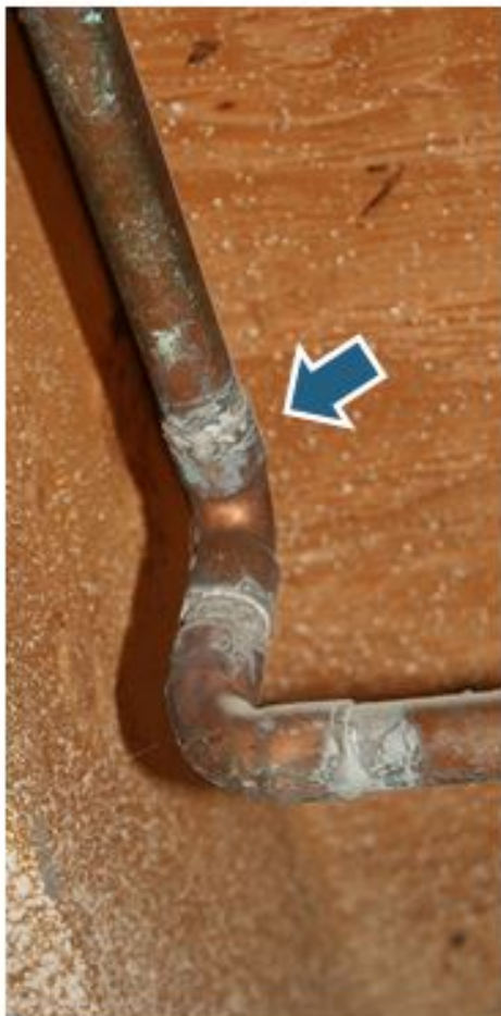
LEAD SOLDER ON COPPER PIPES
