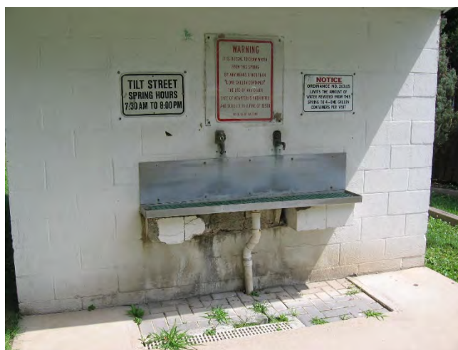
Figure A-84. Two-spigot outlet of Tilt Street Spring. Photo, T. Pallis.
